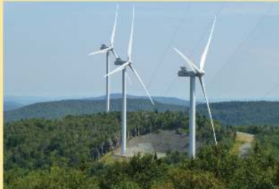
Federal wind tax credits helped Green Mountain Power invest in building a 63 MW wind farm in Lowell, Vermont.
